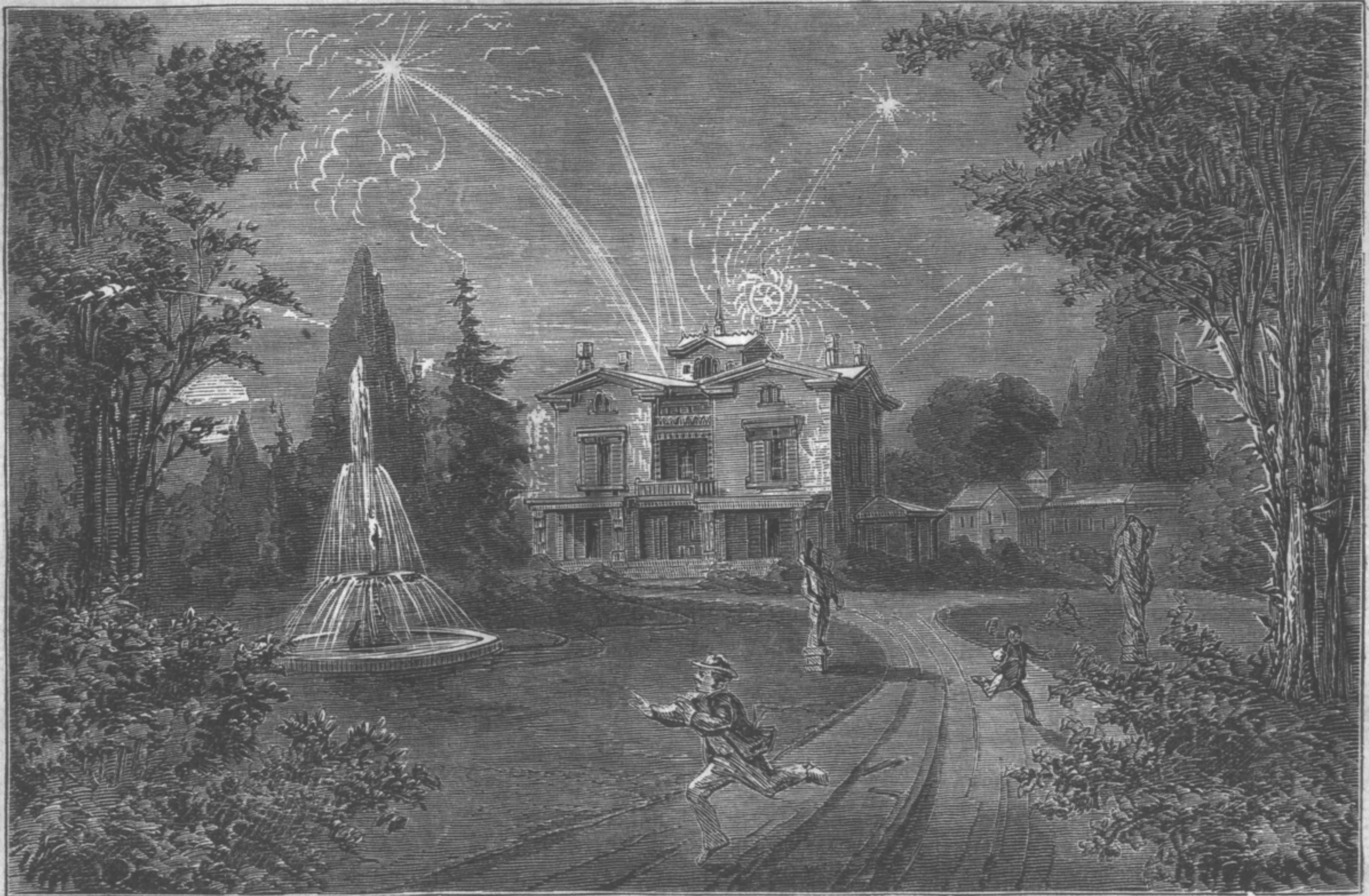
ALARM AT LINDENCROFT.
